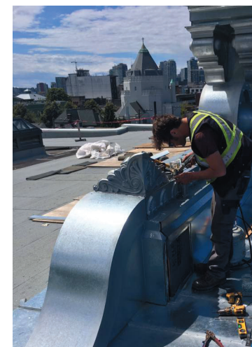
Working on the face of the Tamura Building
